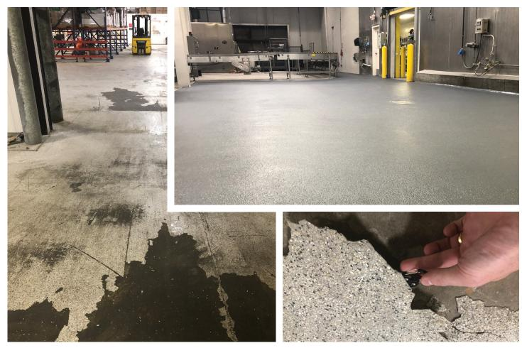
**Problem:** Failing, flaking floor; potential to lose health inspection points
