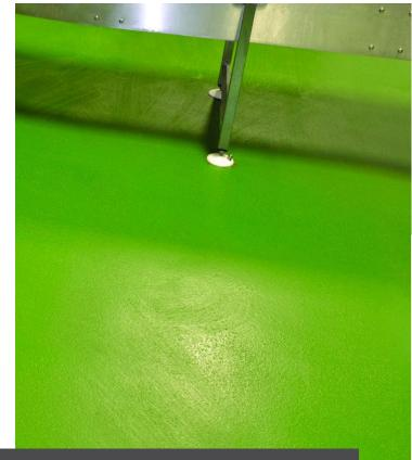
1380m<sup>2</sup> Stonclad UF of co-polymer screed to the desired drainage "falls."
